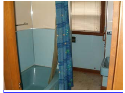
Check plumbing & fixtures
